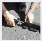
Seamless joining of PAVE EDGE® STARR and PAVE EDGE® STARRFLEX elements using the provided connecting pipes. This does not apply to PAVE EDGE® LIGHT/LIGHTFLEX.
