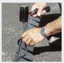
Simple fixing of the *PAVE EDGE*® elements with nails.
